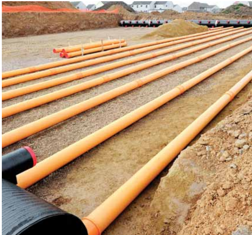
Figure 6.1. Ground to air heat exchanger (REHAU)
