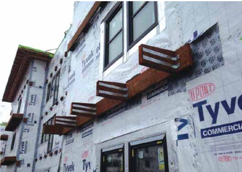
Figure 3.13. Low-tech low-price fixed shades and the way they are mounted, taking into account thermal bridges (Passivehouse Canada)
