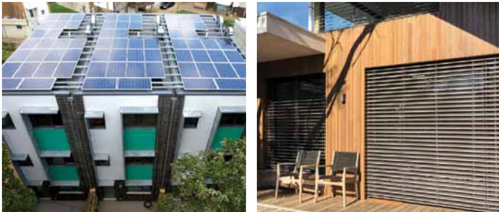
Figure 3.11. Fixed shades on Belfield Townhomes Philadelphia Passive House (left) and motorized venetian blinds (right)
