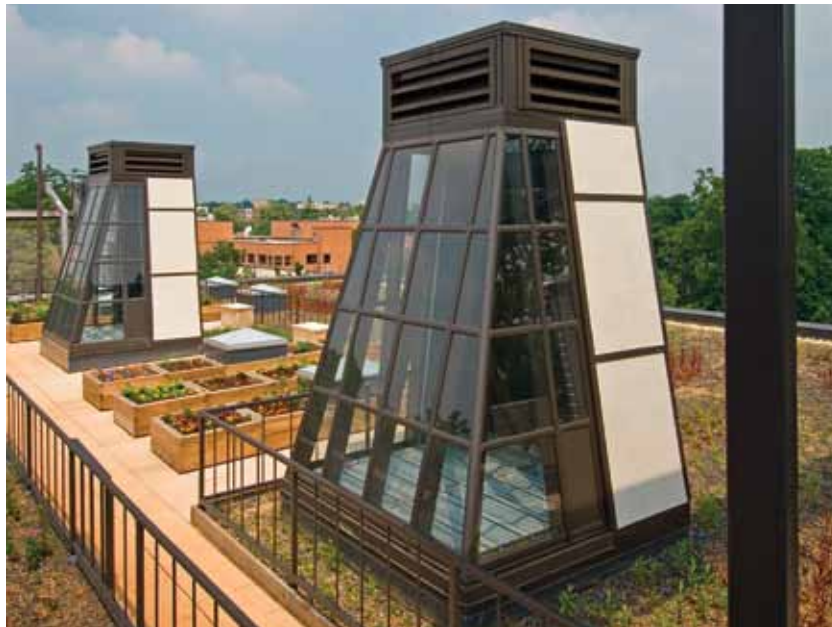
Figure 6.4. A solar chimney(s) as a way to increase draft needed for passive cooling
